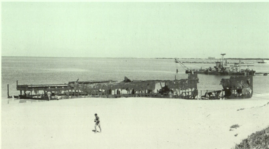
Figure 8 The Alacrity during dredging activity. Photo: Jon Carpenter.
