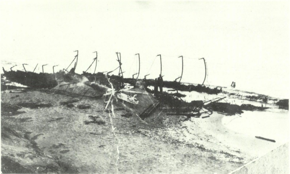
Figure 11(a), (b) The burnt-out remains of the Abemama showing exposed deck supports. Photos: Mrs McGhie
