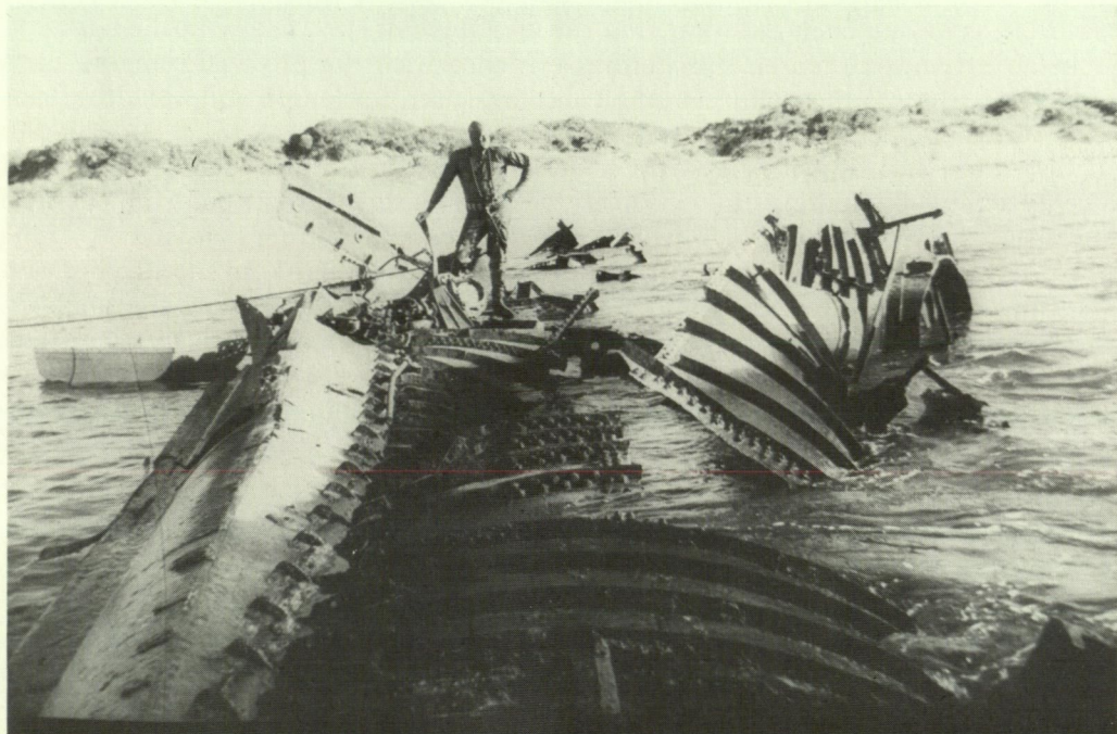
Figure 3 K VIII in the early stages of demolition. Sullivan Collection.
